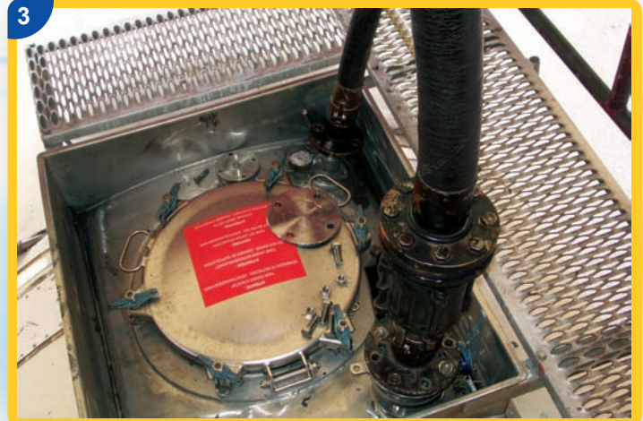
Filling the bulk container by means of a gas balance line in a chemical plant in Spain.
